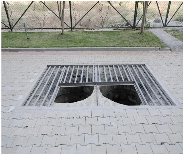
Rain water Recharge Pit
