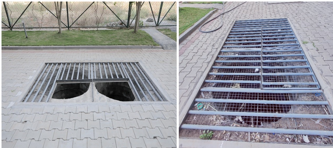
Rain water Recharge Pit
